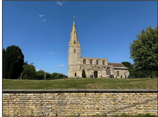
Plate 9: View of St. Peters Church from Church Street.
