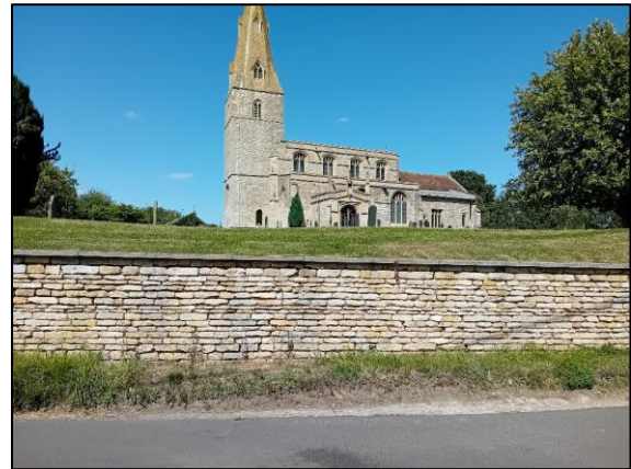
Plate 16: Church wall recently repaired. Some areas still need cleaning of vegetation.
