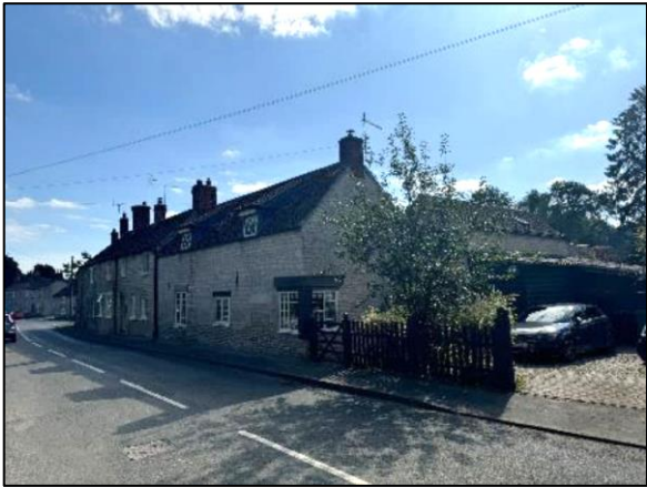
Plate 7: 35 High Street, remnants of the original lower roofline visible on gable end.
