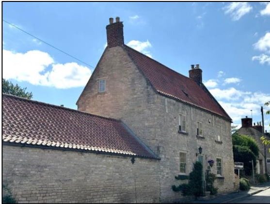
Plate 12: No 1 Chapel Hill, also referred to as Manor House.
