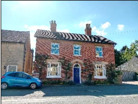
Plate 4: No.15 High Street, made of brick which is fairly unique to the conservation area, but it is unfortunate that the 1 st floor windows have been replaced with uPVC.
